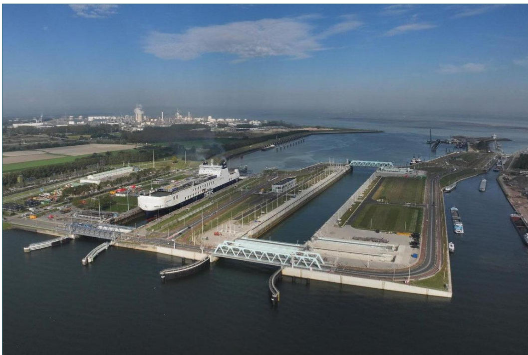
Figure 4-18: Lock 'Nieuwe Sluis Terneuzen' in Terneuzen, the Netherlands 26
