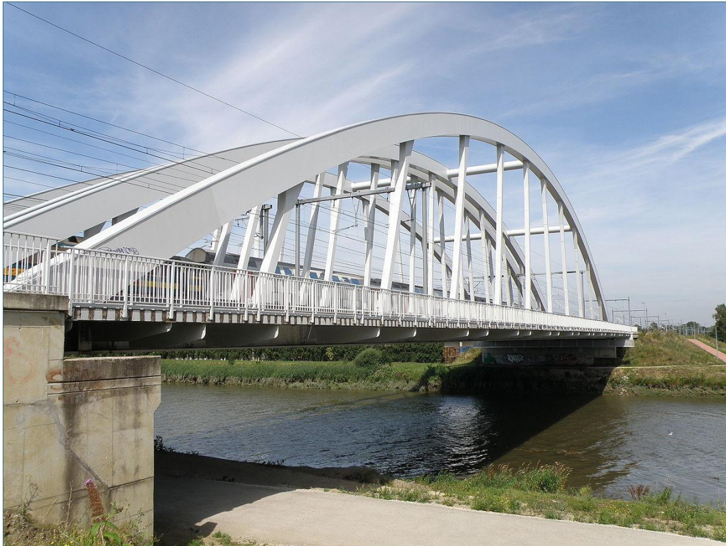
Figure 4-23: Fixed bridge 'Spoorbrug' in Duffel, Belgium 33
