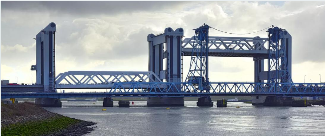
Figure 4-25: Vertical lift bridge 'Botlekbrug' in Rotterdam, the Netherlands 35,36
