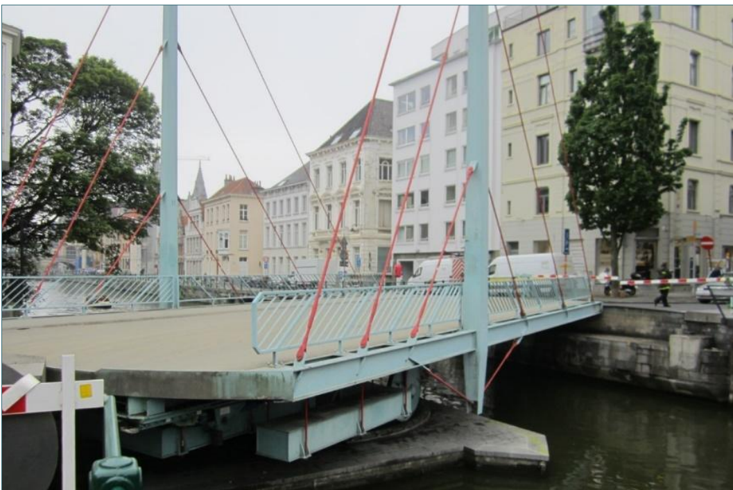
Figure 4-26: Swing bridge 'Predikherenbrug' in Ghent, Belgium 37,38
