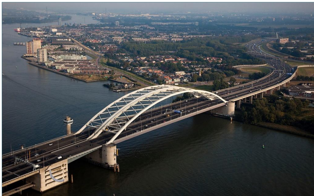
Figure 4-24: Fixed bridge 'Van Brienoordbrug' in Rotterdam, the Netherlands 34
