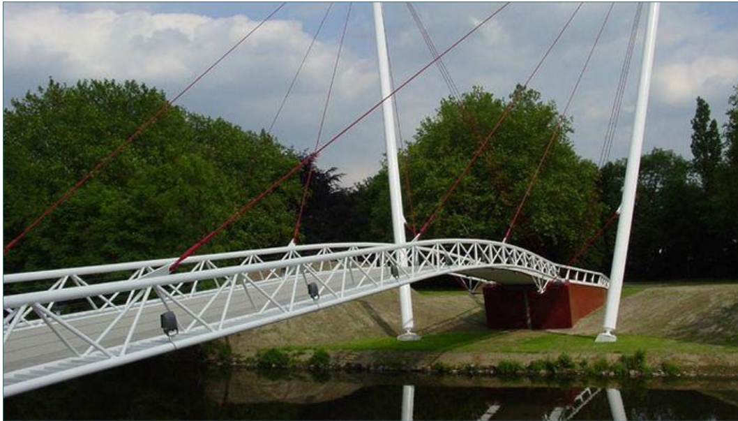
Figure 4-27: Suspension bridge 'Ledeberg Leeft' in Ghent, Belgium 39
